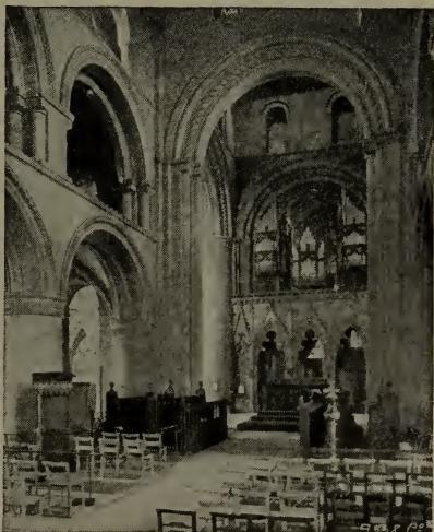
NAVE, LOOKING EAST.
